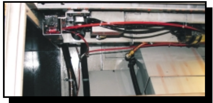
Red Firetrace Detection Tubing Routed Throughout The Machine, Cooper Discharge Piping And Silver Discharge Nozzles At The Top
