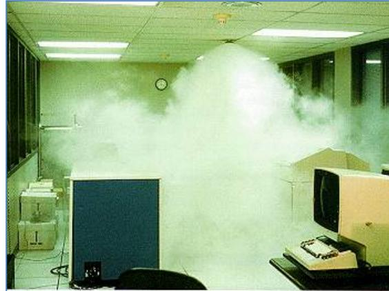
Figure 1: Clean Agent discharge causes cooling due to decompression.
