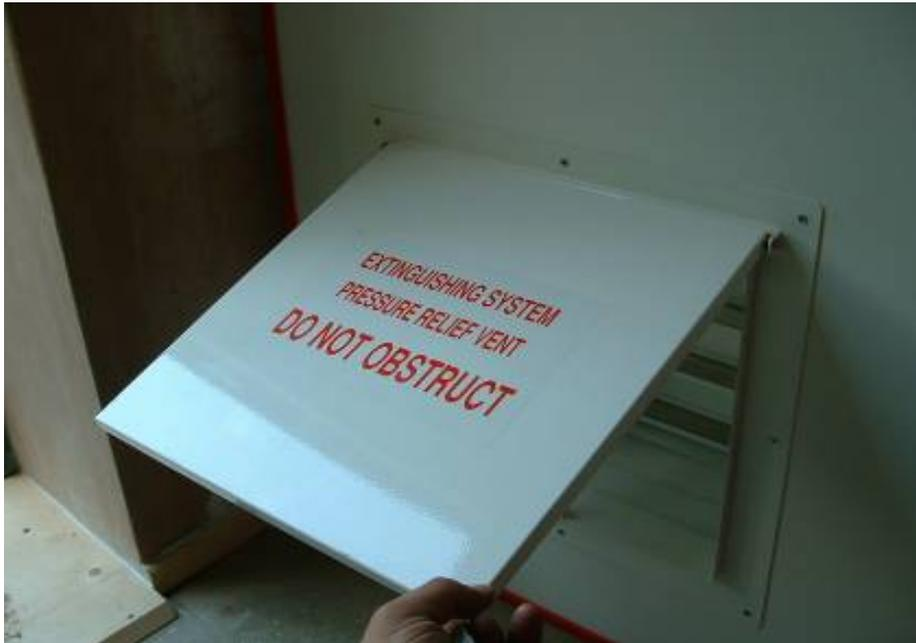
Figure 11: the sign says "DO NOT OBSTRUCT", because it is very likely the vent path will be obstructed which is why the vent path must be checked regularly.
